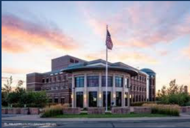
Missouri River Federal Courthouse Great Falls, MT
